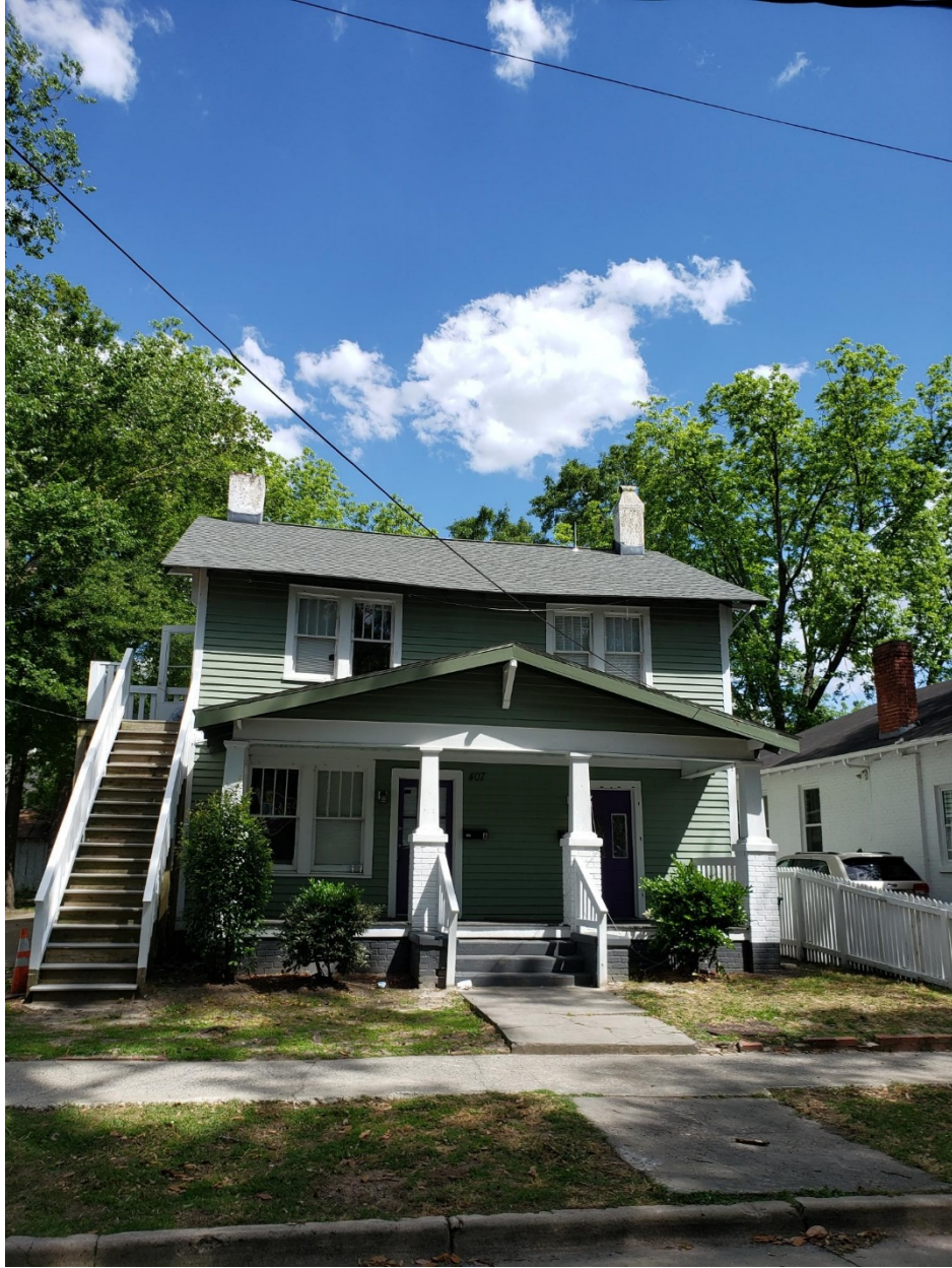
2021-23 407 S. Jarvis Street Replace shingles with like color
