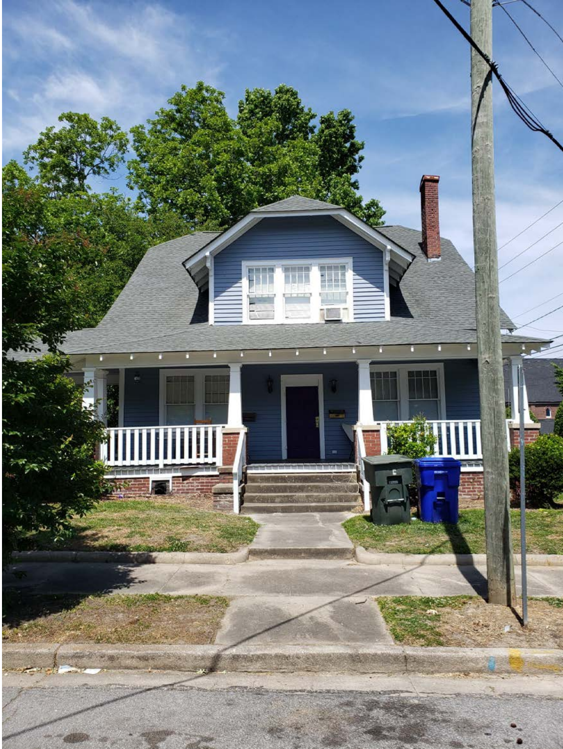
2021-25 400 S. Holly Street Replace shingles with like color
