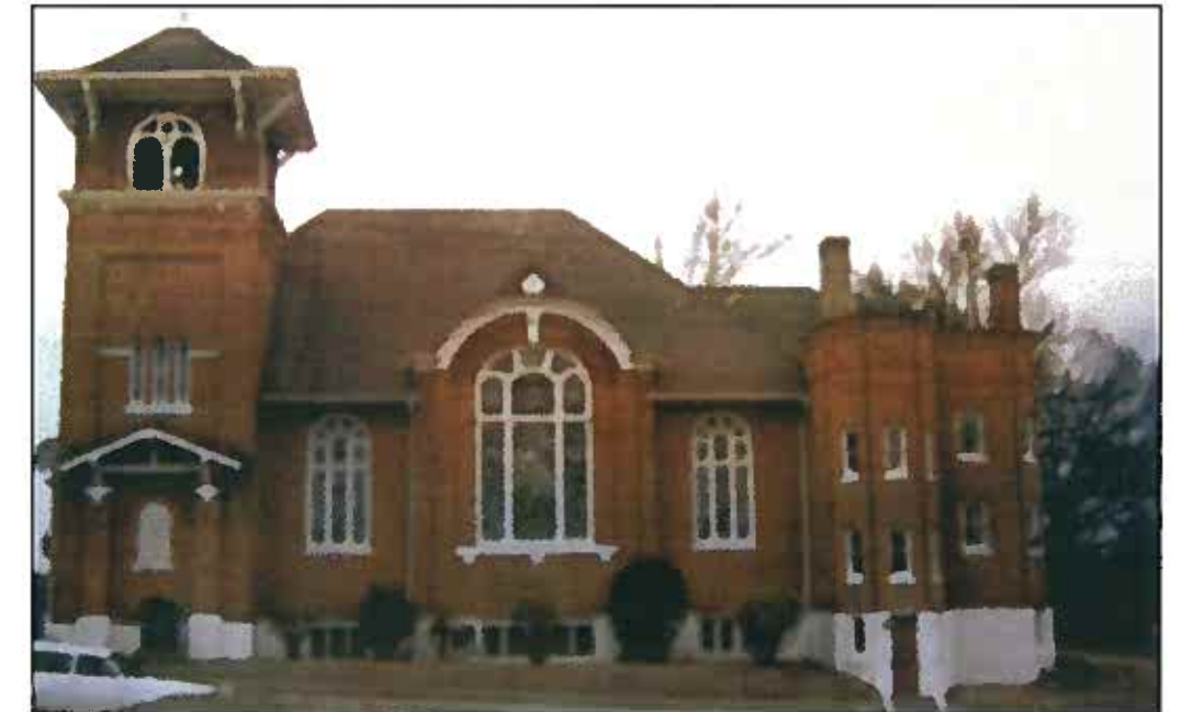
Archieve photo of Sycamore Hill Baptist Church's bell tower.
