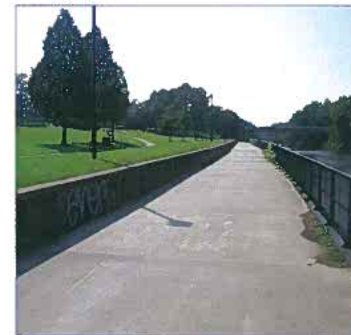
Walkway Along Bulkhead
