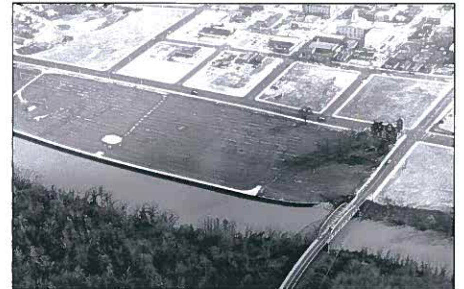
The Town Common site after clearance with only the Sycamore Hill Baptist Church remaining in the top right corner of the photo.
