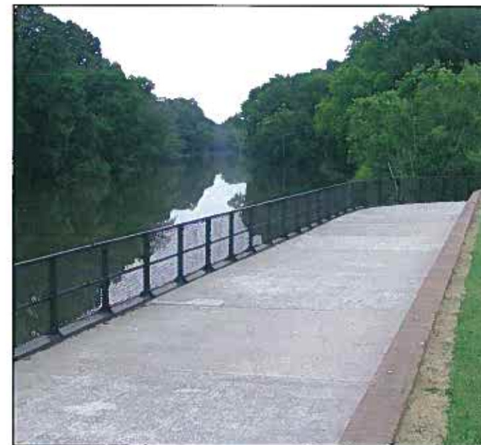
Walkway Along Bulkhead
