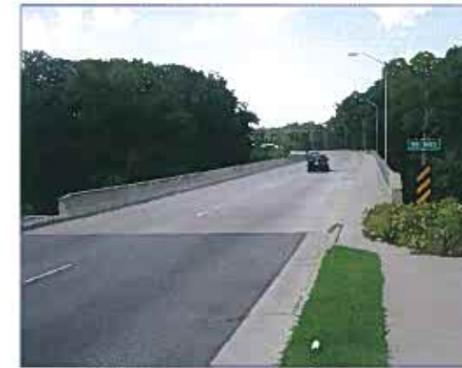
Greene Street Bridge
