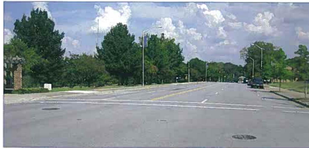
First Street - Looking East
