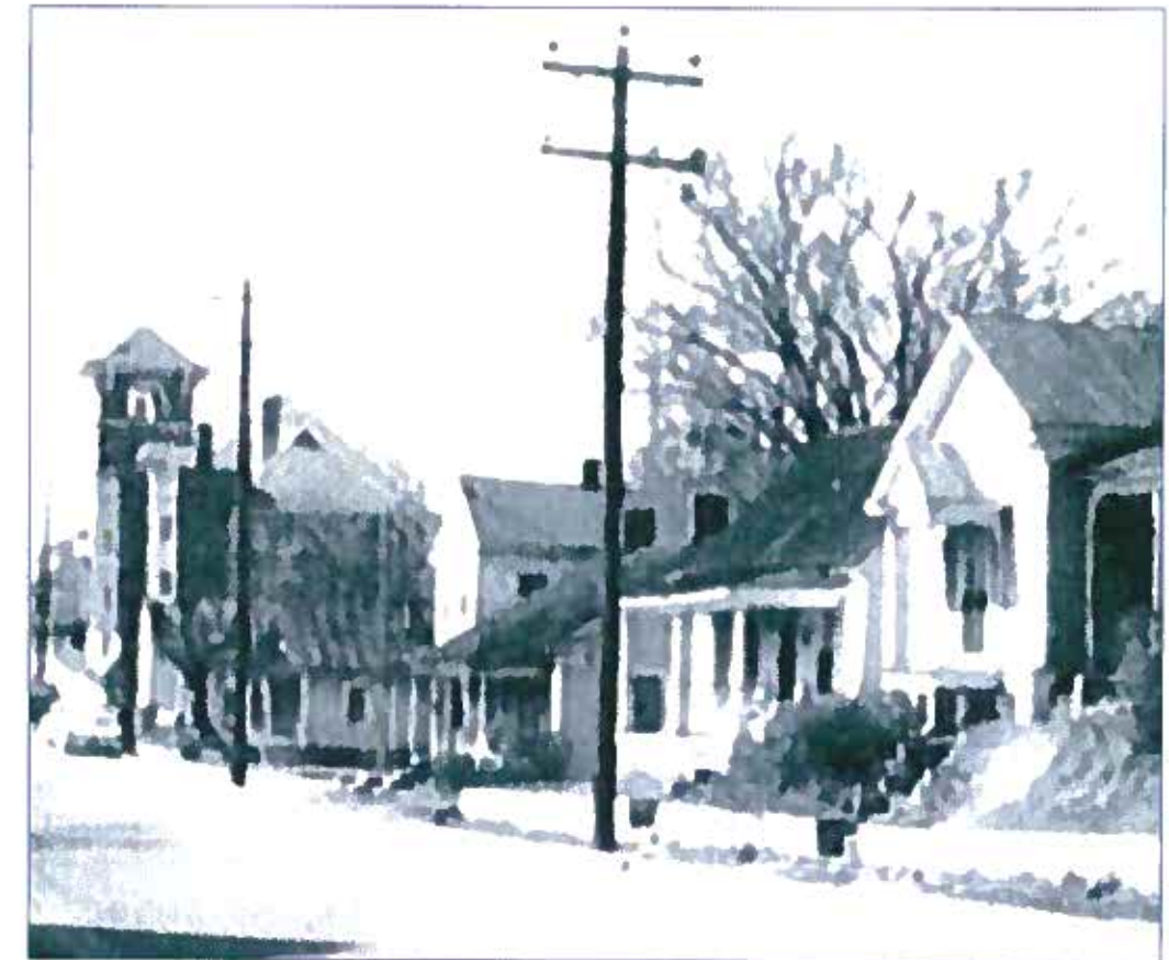
View down First Street showing the church in the background.
