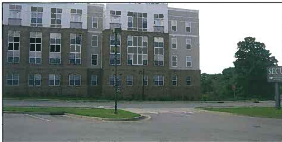
Recent private development adjacent to the Town Common
