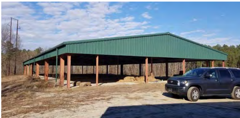
Three existing metal roofed buildings offer great potential for a variety of uses from office, recreation programming, or leasable space.
