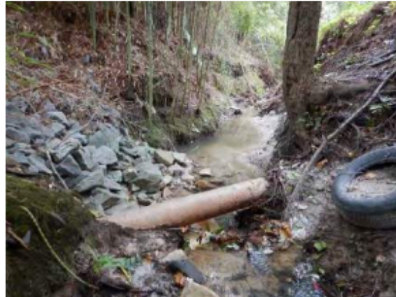
Picture 5-11: Exposed Gravity Sewer Crossing
