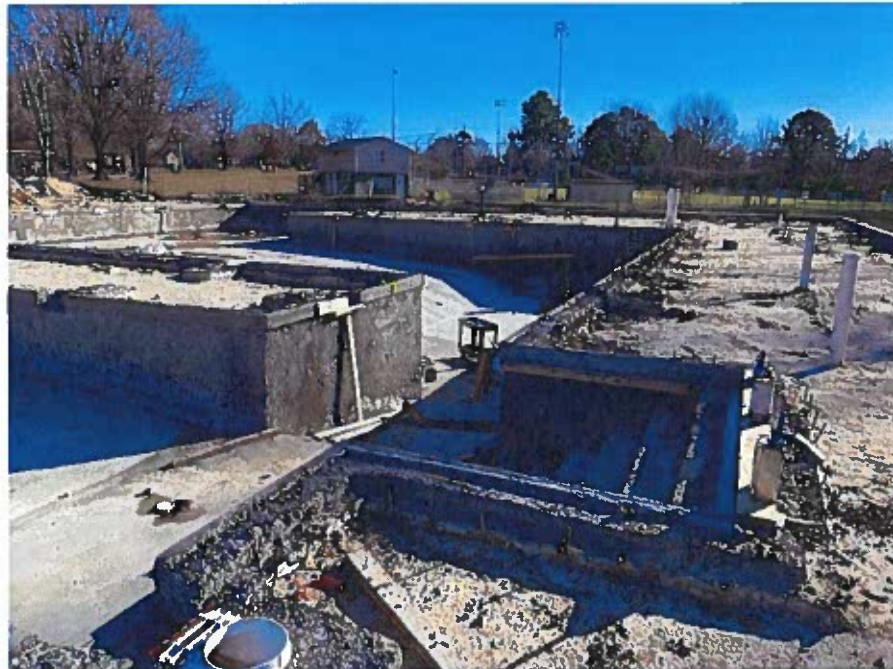
Outdoor Pool Construction
