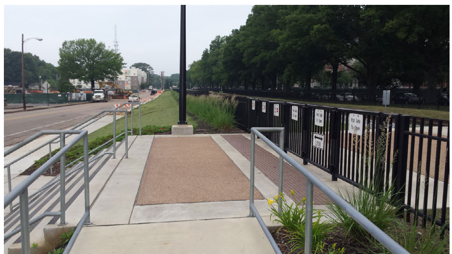
This pedestrian rail crossing at the University of Memphis uses pull gates to encourage pedestrians to look for trains before crossing the tracks. The exit gates to the left of the entrance gates prevent pedestrians from getting caught on the tracks.
