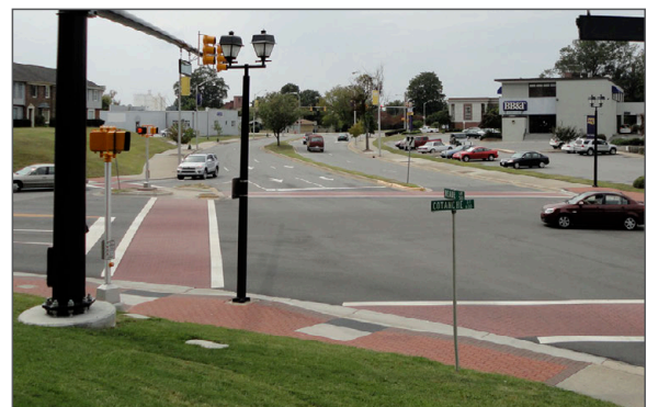
Intersection of Cotanche St and Reade Cir, with brick crosswalks.
