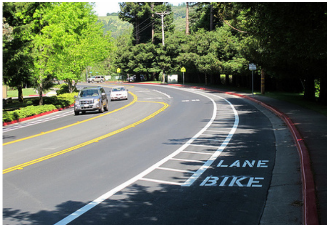
The use of pavement markings delineates space for cyclists to ride in a comfortable facility.
