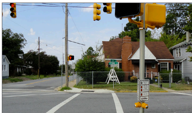
Intersection of 14 St & Fleming St, with crosswalks, curb ramps, and countdown signals.
