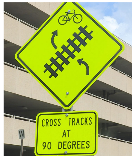
Signage can be used to reinforce the risk at skewed rail crossings and guide cyclists to cross tracks at 90 degrees.
