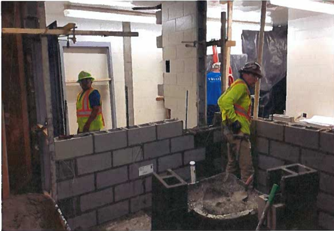
Family Restroom Construction at the Greenville Aquatics and Fitness Center
