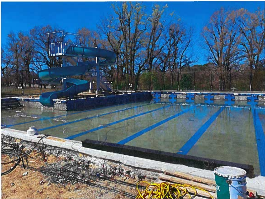
Outdoor Pool Construction
