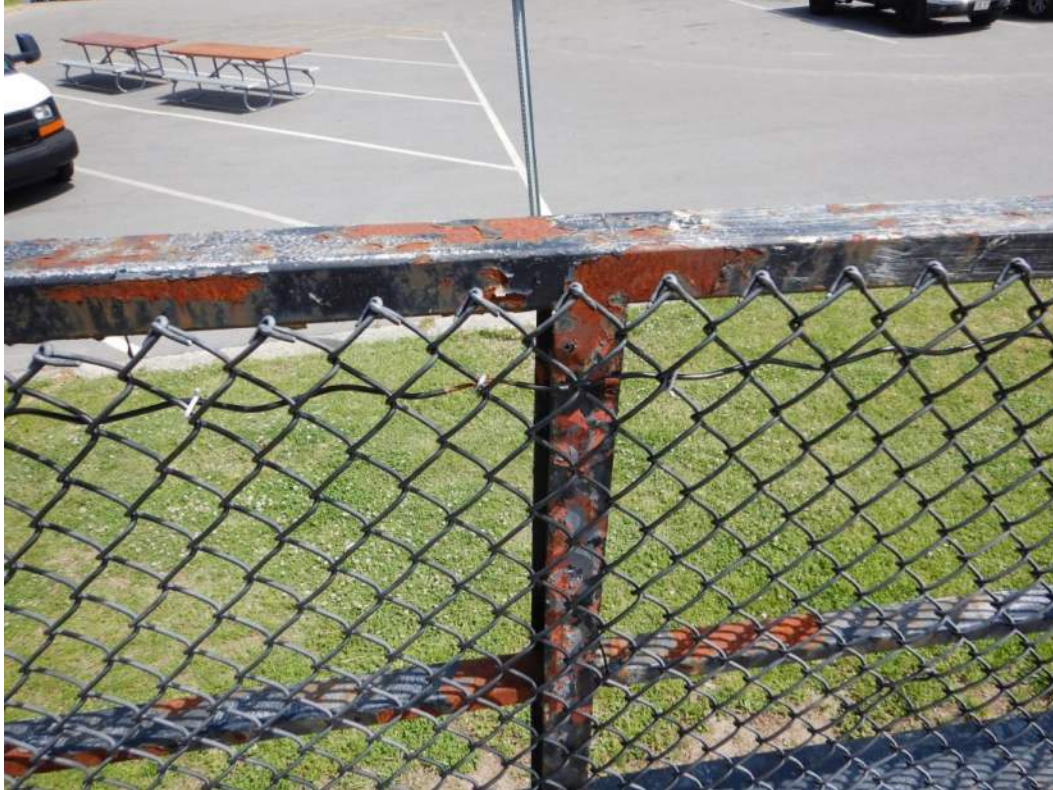
PHOTOGRAPH 2.3: TYPICAL CONDITION OF EXISTING HANDRAIL
