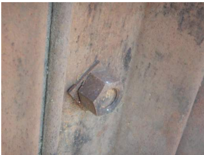
PHOTOGRAPH 2.5: TIE ROD NUT
