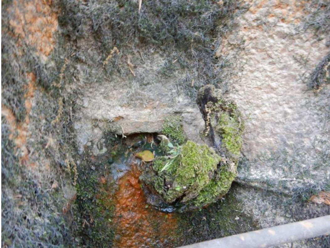
PHOTOGRAPH 2.6: TYPICAL CONDITION OF SHEET PILE WEEP HOLES
