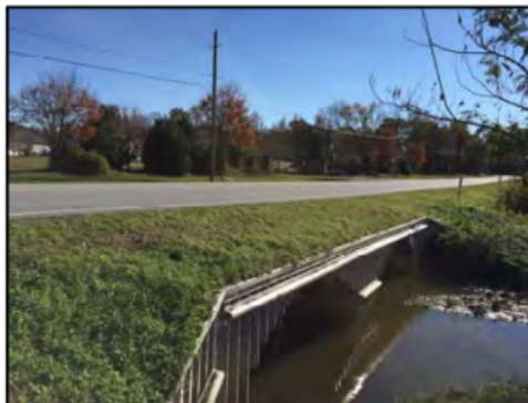
Picture 4-3. Corey Road CMP arches
