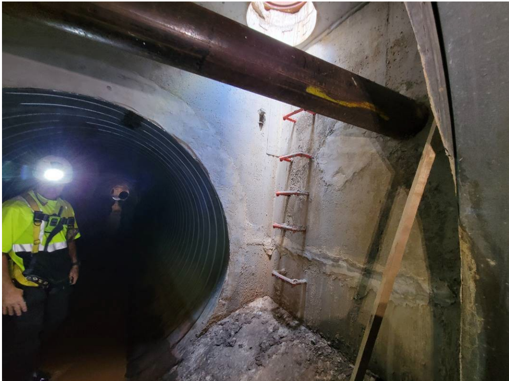
Photo 32 Sta 14+36 Manhole with water line
