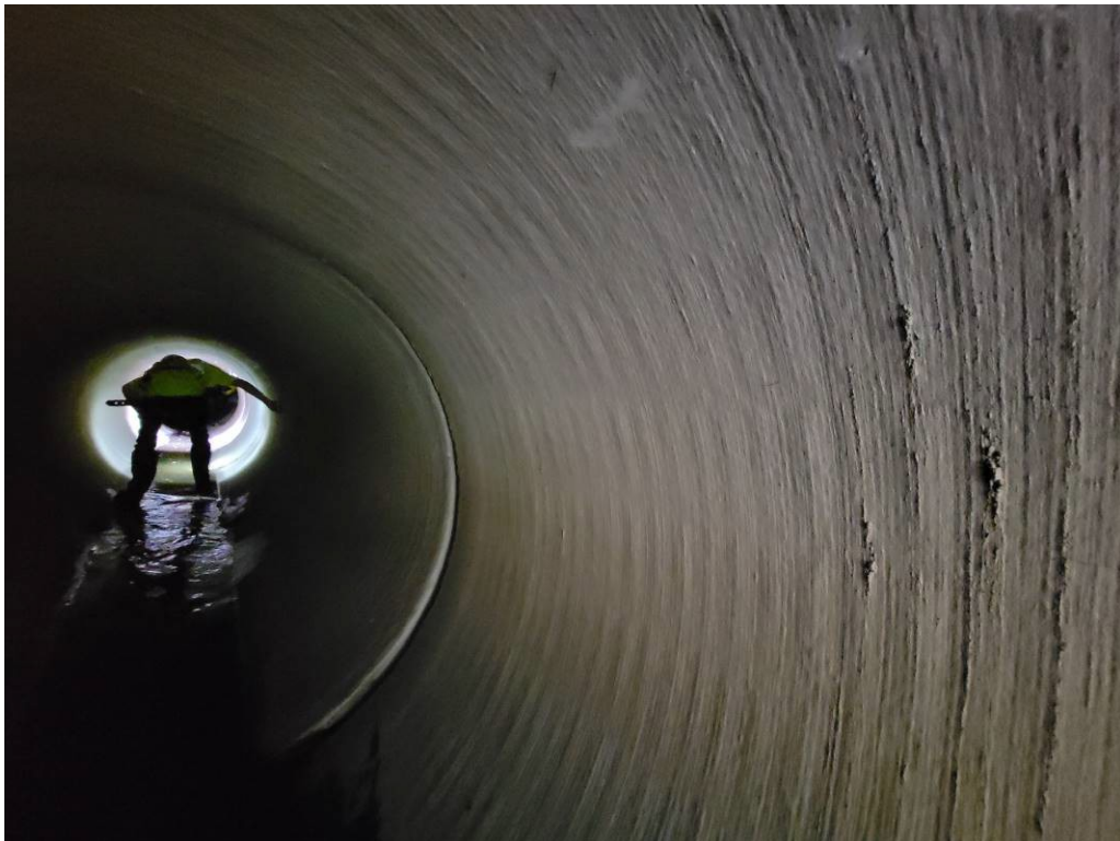
Photo 2 Precast RCP at Skinner
