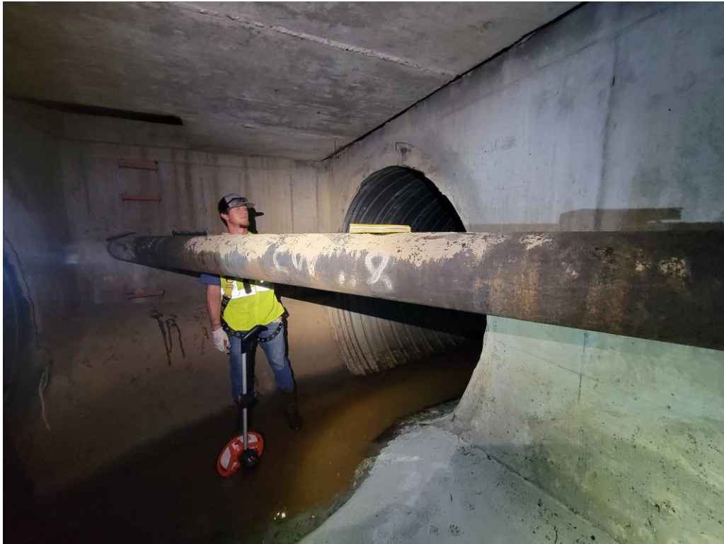
Photo 15 Sta 4+88 Manhole with water line
