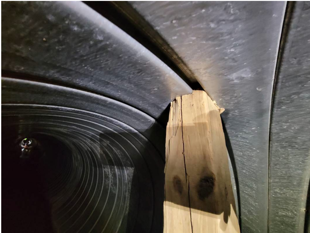
Photo 36 Top of 4x4 post. Appears contoured to fit flutes
