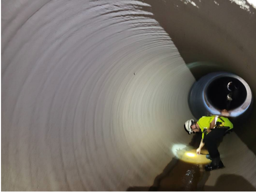
Photo 21 Spray liner from sta 7+33 to 7+61
