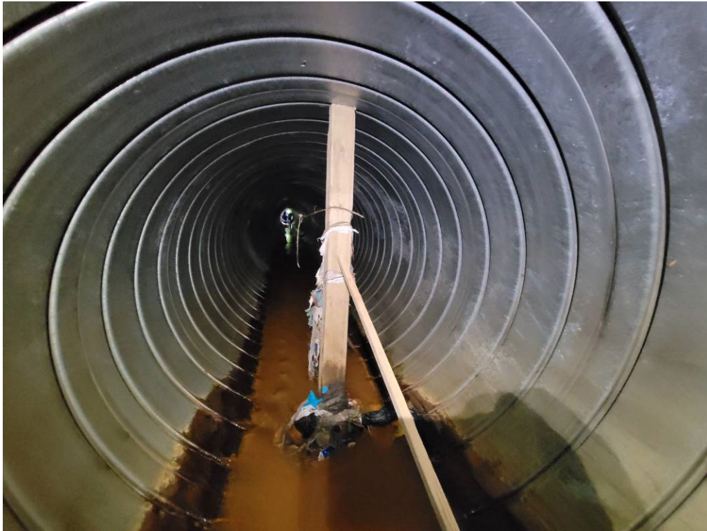
Photo 35 Sta 15+75 4x4 post in 54" pipe
