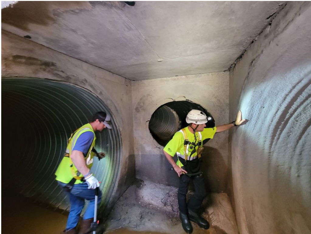
Photo 20 Sta 7+33 Manhole at spray liner trial
