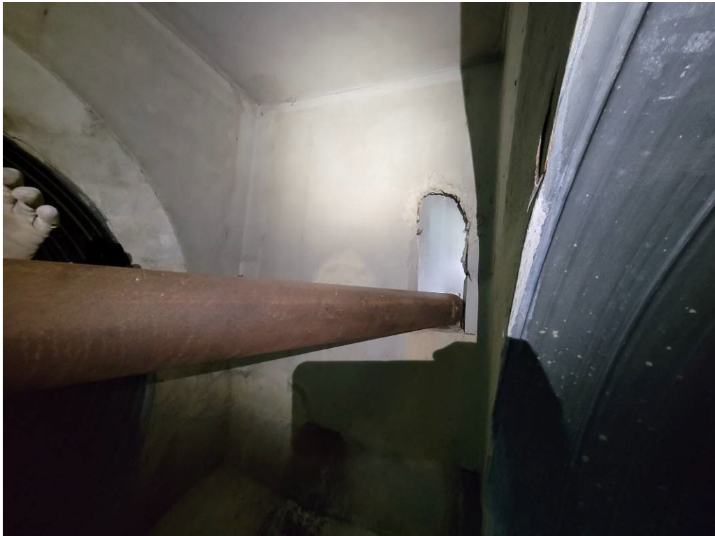
Photo 28 Sta 11+11 Manhole with water line
