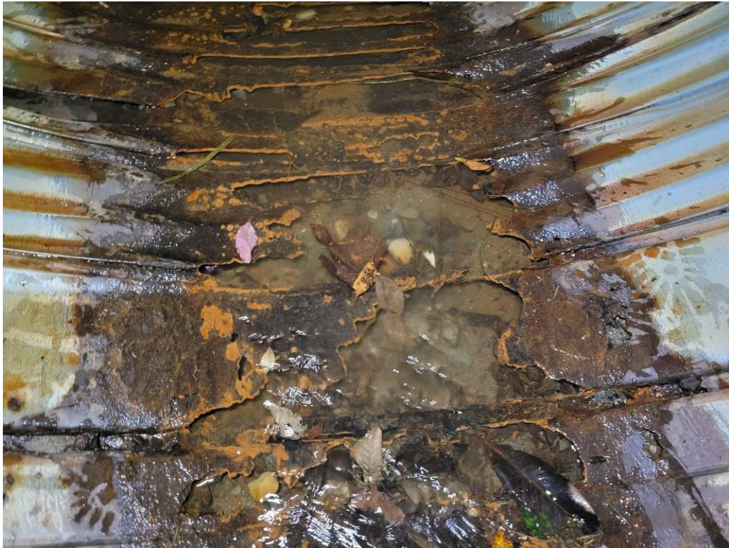
Photo 9 CSP below water line, typ sta 0 to 1+90
