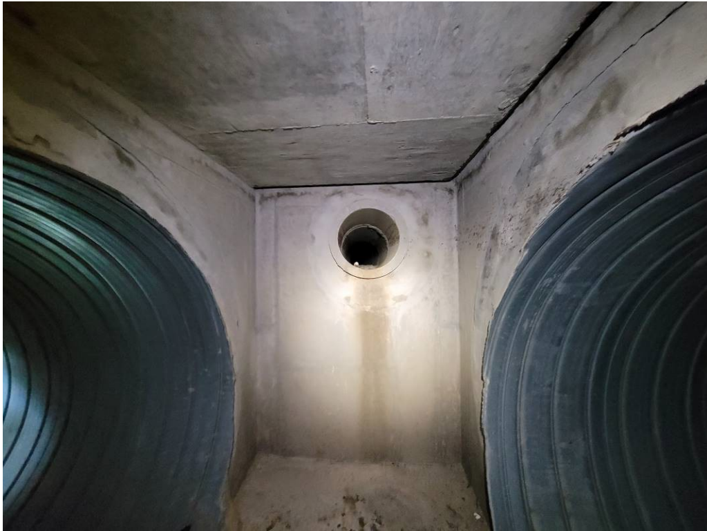
Photo 17 Sta 6+00 Manhole with 24" lateral
