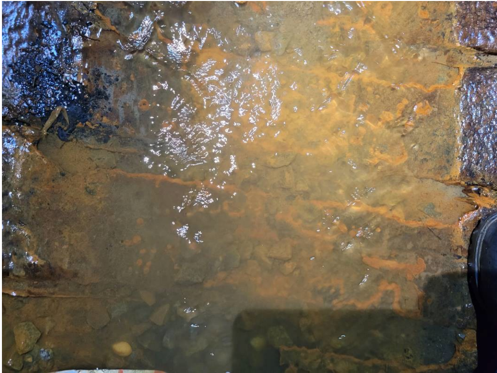
Photo 25 Sta 9+46 Severe corrosion. Sample of soil attempted
