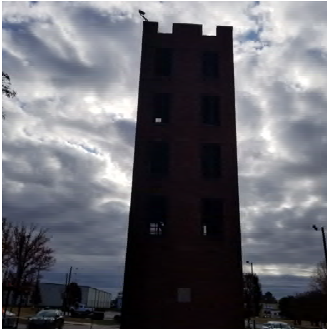
PHOTOGRAPH NO. 2: OVERALL REAR VIEW
