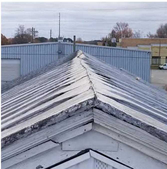
PHOTOGRAPH NO. 28: ROOF RIDGE AND GABLE END
