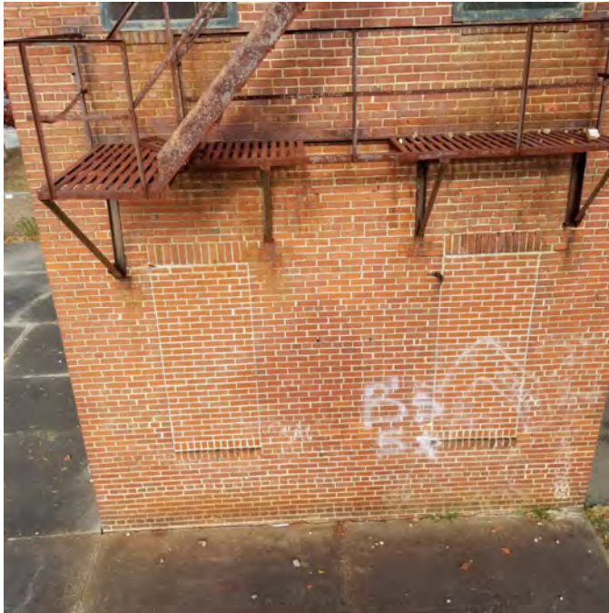
PHOTOGRAPH NO. 8: FRONT VIEW 1 ST FLOOR
