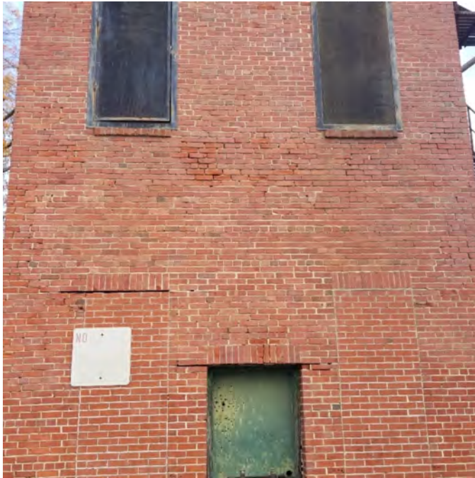
PHOTOGRAPH NO. 12: SIDE VIEW 1 ST FLOOR
