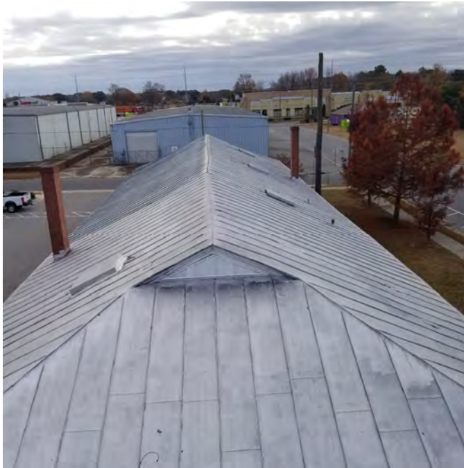
PHOTOGRAPH NO. 27: OVERALL VIEW OF ROOF
