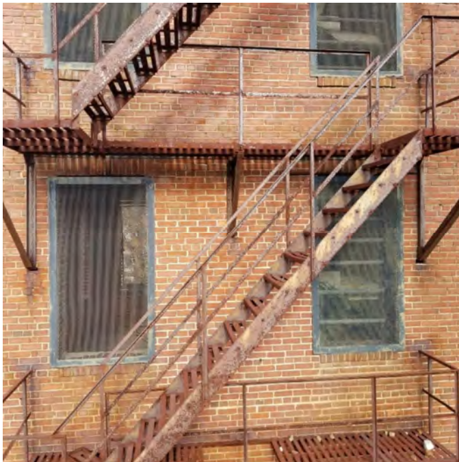
PHOTOGRAPH NO. 7: FRONT VIEW 2 ND FLOOR
