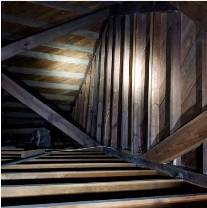
PHOTOGRAPH NO. 33: WALL FRAMING AT ROOF GABLE END
