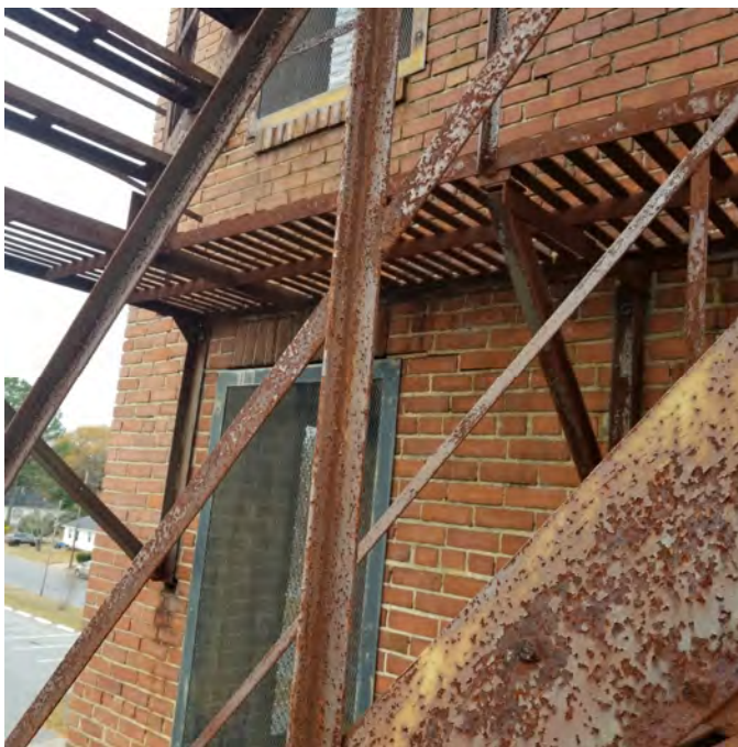
PHOTOGRAPH NO. 13: EXTERIOR STAIR
