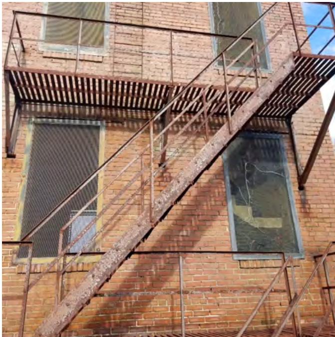
PHOTOGRAPH NO. 5: FRONT VIEW 4 TH FLOOR
