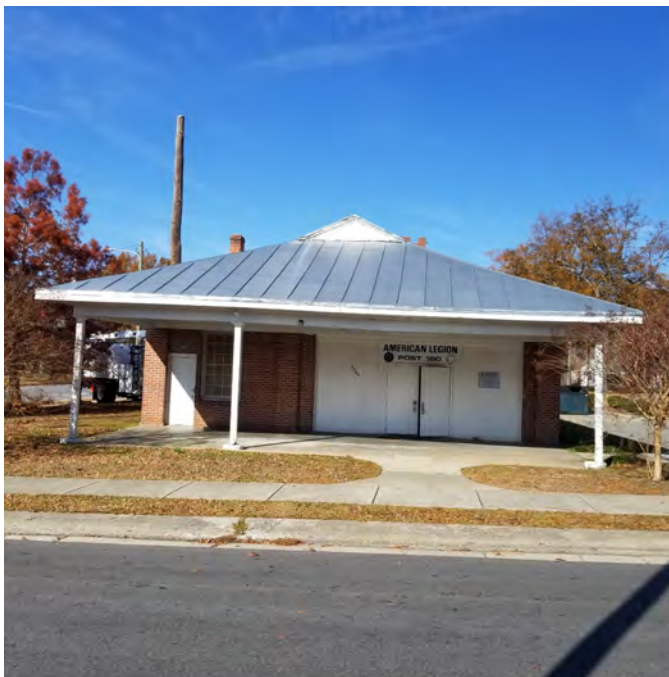
PHOTOGRAPH NO. 24: EXTERIOR FRONT VIEW
