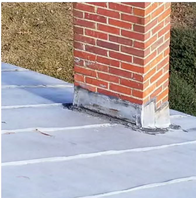
PHOTOGRAPH NO. 32: FLASHING AT CHIMNEY
