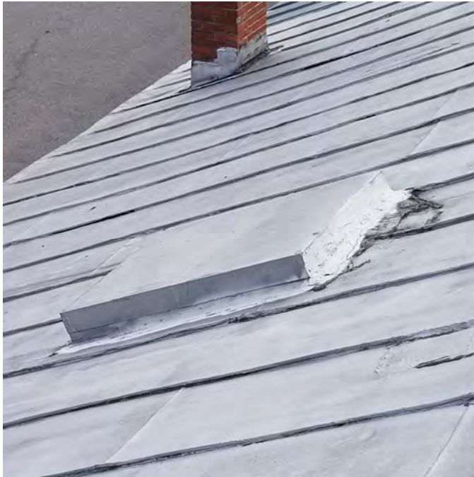
PHOTOGRAPH NO. 29: COVERED SKYLIGHT
