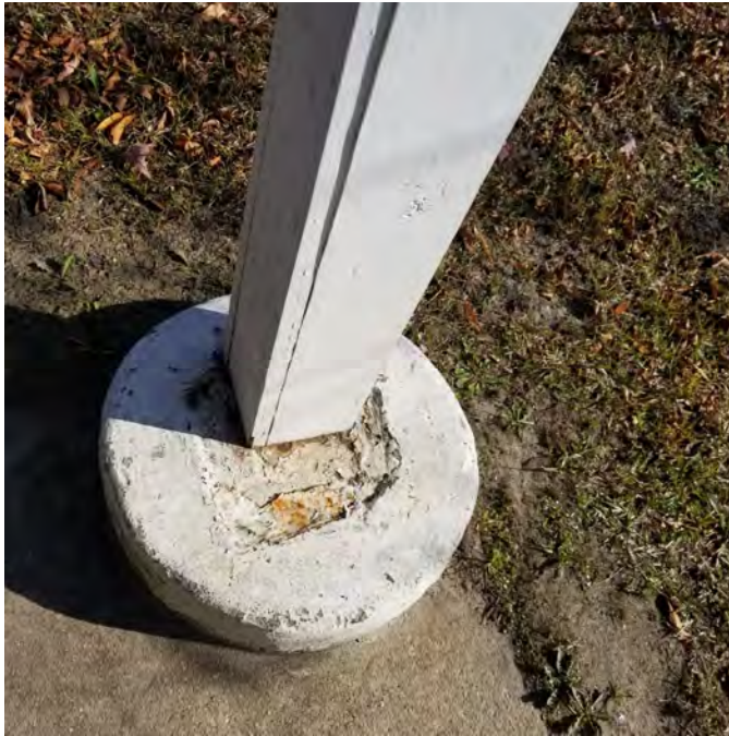
PHOTOGRAPH NO. 35: REPLACED ENTRY COLUMN
