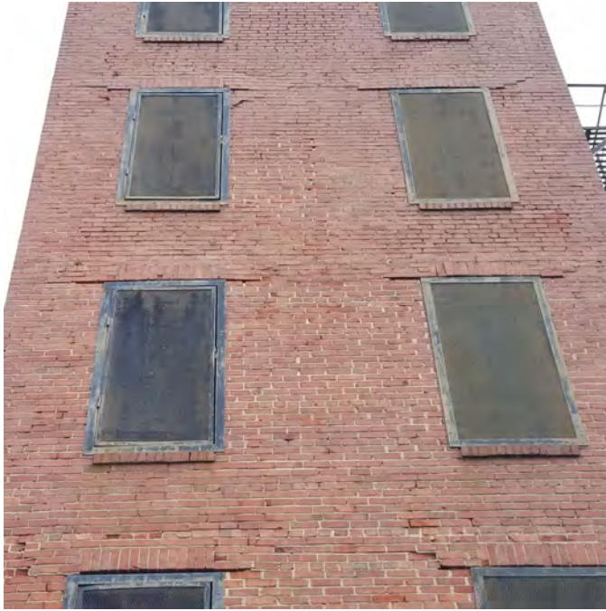
PHOTOGRAPH NO. 10: SIDE VIEW 3 RD FLOOR
