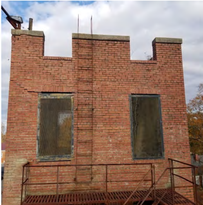
PHOTOGRAPH NO. 4: FRONT VIEW 5 TH FLOOR
