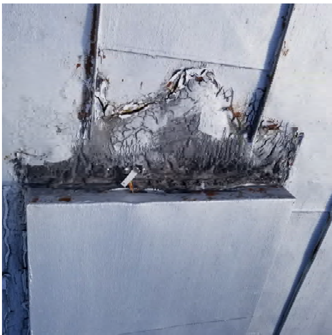
PHOTOGRAPH NO. 30: ROOF FLASHING AT COVERED SKYLIGHT
