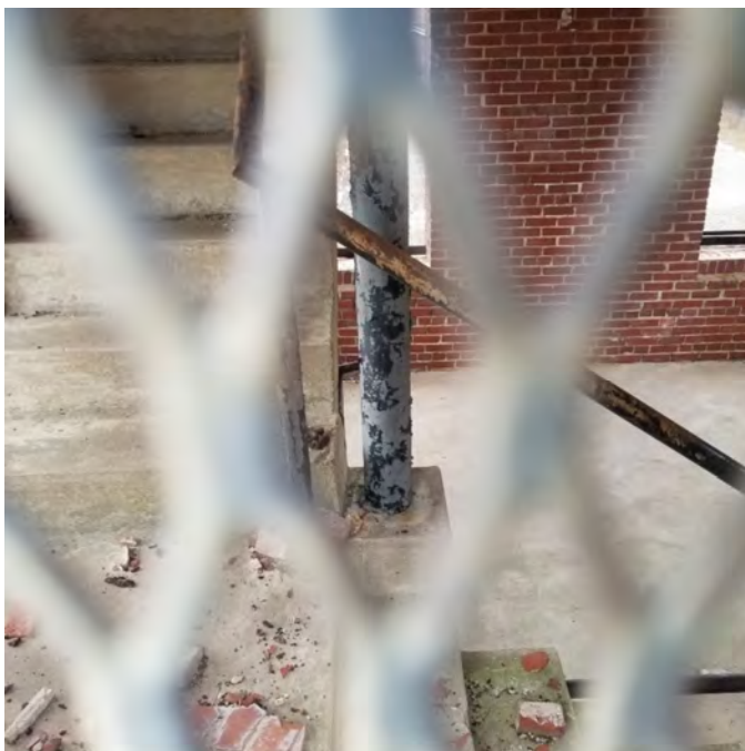
PHOTOGRAPH NO. 23: INTERIOR FIRE POLE
