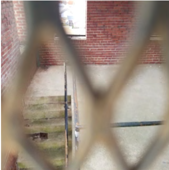
PHOTOGRAPH NO. 22: INTERIOR VIEW OF STAIRS/LANDING
