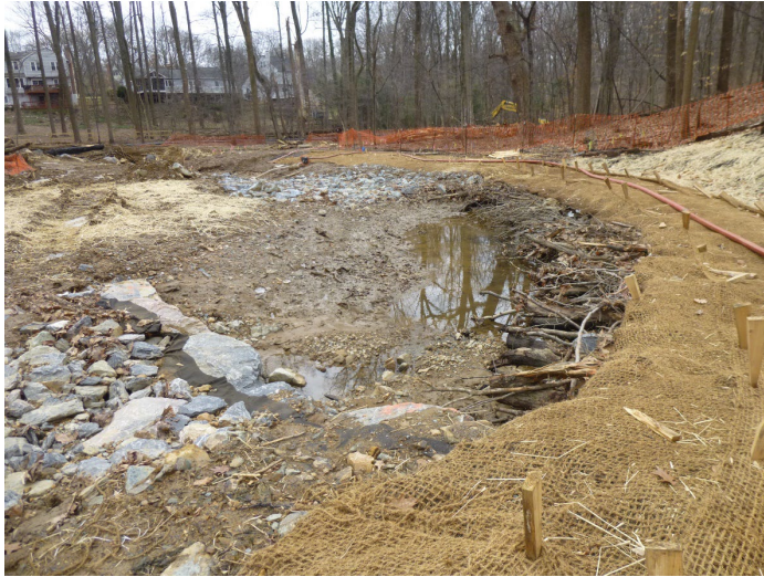
Bank grading and coir mat for flatter bank slopes
