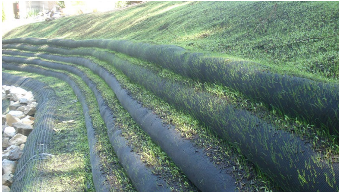
Bank grading with a geotextile support for moderate to steep banks
