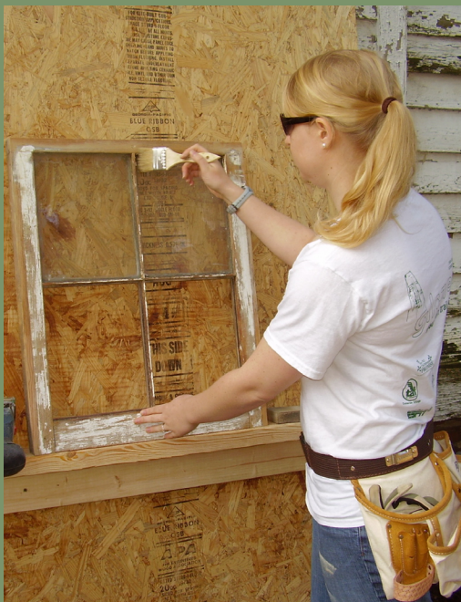
A student in the Edgewcombe Community College Preservation Trades Program primes a window sash during the restoration process. Photograph courtesy Monika Fleming.
