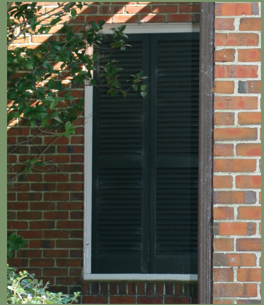
Closed shutters effectively block out solar radiation while louvers can still allow ventilation.
