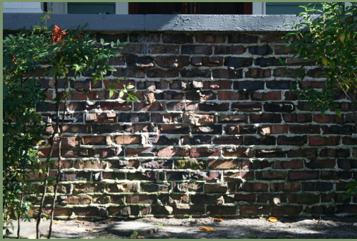
Skintled brickwork is one of the distinctive exterior wall materials found in the College View Historic District.
