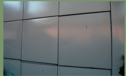
The porcelain-enameled-steel panels as seen above are a defining element of the iconic Lustron house.
