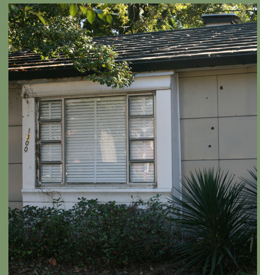
Aluminum casement windows in the Lustron house.
