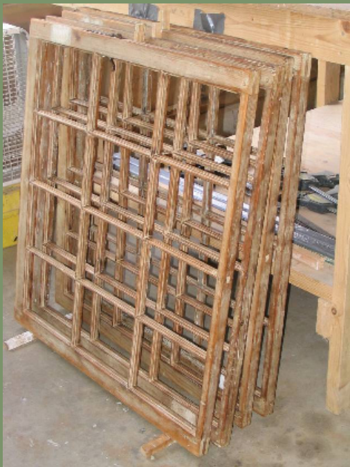
Window sash stripped of their paint by use of steam sit ready for replacement of their glass. It is not always necessary to strip a window for restoration work, but if extensive wood repairs are necessary or lead abatement is desired, steam is a good method for paint removal.
