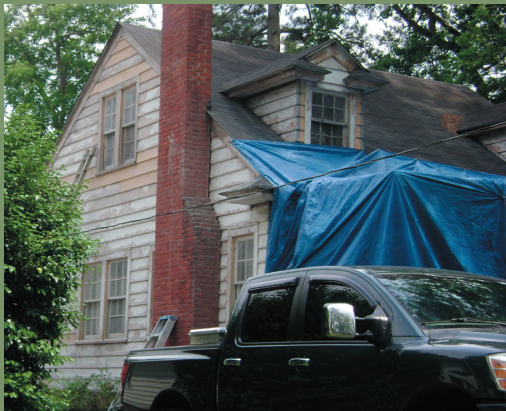
Original weatherboards are scraped and prepped for painting during restoration.
