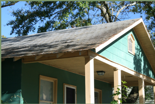
Original pressed tin shingles cover a College View Historic District roof.
