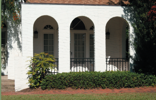
Although most of Greenville’s local landmark and historic district porches are primarily wood, some like the two above examples also feature brickwork, stucco and ironwork.
