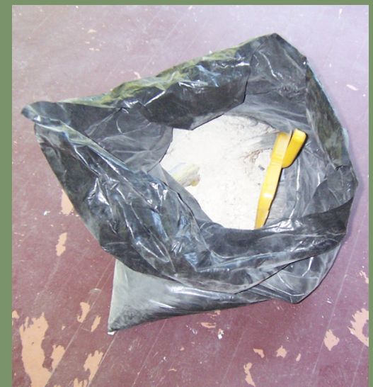
Paint scrapings should always be contained during work and collected and properly disposed of in a heavy trash bag. Bags should be closed by twisting the top, folding it down in a gooseneck, and securing it with duct tape.
