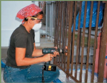
Prepping ironwork for painting with a wire brush drill attachment.
