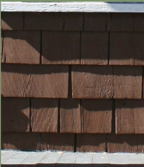
Sunlight highlights the textural character of wood shingles on a bungalow in the College View Historic District.
