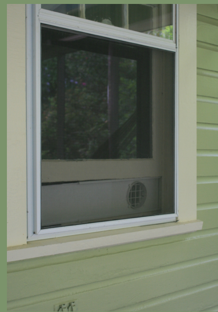
The vent of a portable air conditioning unit is far less obtrusive and less damaging to the window fabric than a window unit.
