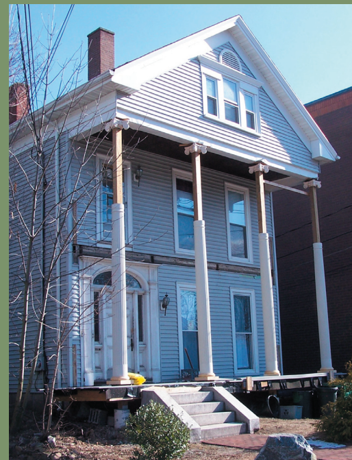
These precast columns demonstrate just how bad the results can be when imitation features literally fall short of original historic fabric. When replacement of an element is necessary, it must always match the original as closely as possible. Custom work is most often the best way to accomplish the job correctly and with durable materials.
