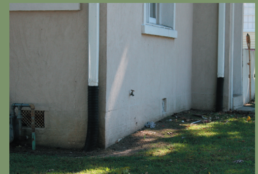
Flexible drains buried in the ground is one effective way to channel water away from a foundation.
