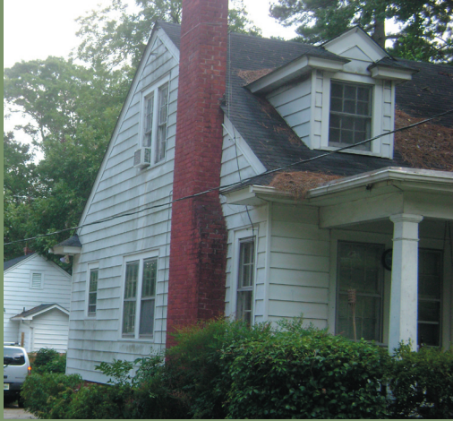
House covered in aluminum siding before project.
