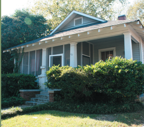
This partially screened porches offers a good example of historically appropriate porch screening. Here, slender wooden uprights support the screening between the boxed columns, which remain prominent and character defining.
