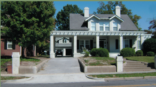
A proposal sketch and after photograph show how a historic concrete retaining wall was successfully preserved while the driveway was widened for improved safety and ease of entry and exit of off busy 5th Street in this COA project.
