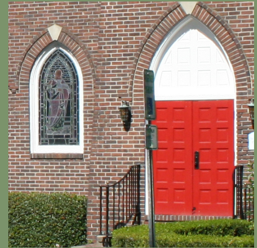
Lancet arched doorway and window with stained glass at St. Paul’s Episcopal Church.
