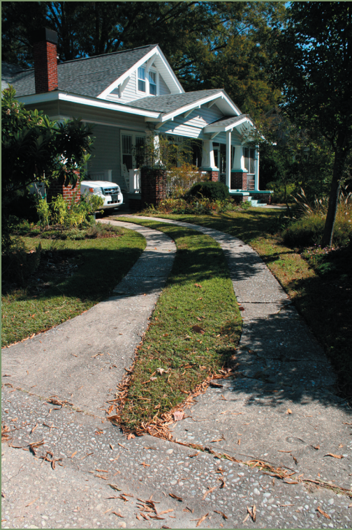
A historic driveway design worthy of emulation. It is not only period appropriate, but its permeability makes it a sound choice for water rainwater management and conservation.
