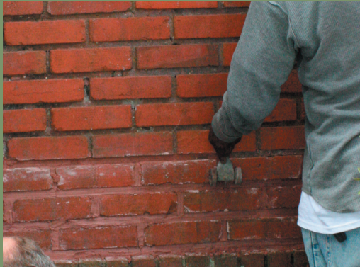
Raking the repointed joints of the above project with a skate.
