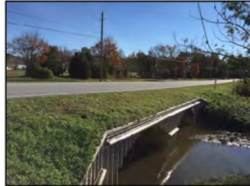
Figure 5. Corey Rd CMP arches
