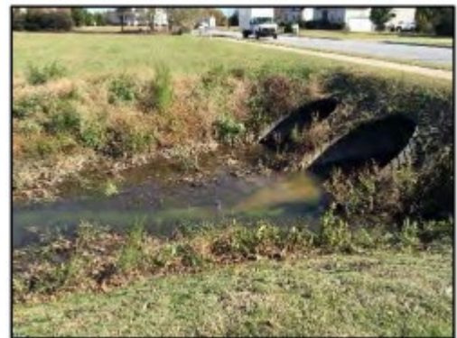
Figure 5. Trafalgar Drive – South Culverts
