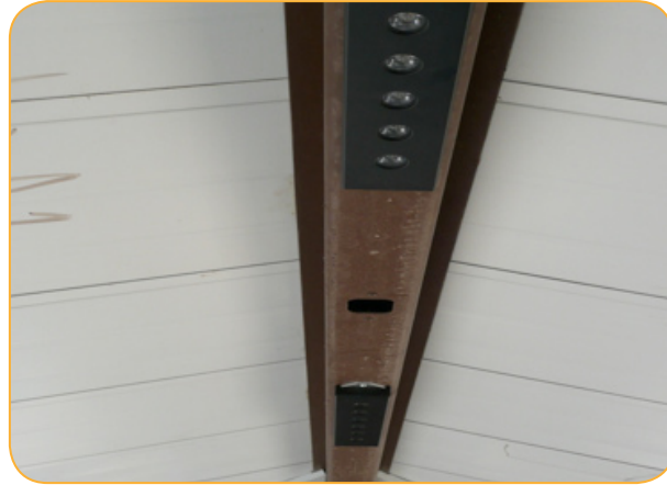
figure 6. Strip luminaire – mounted on ceiling beam
