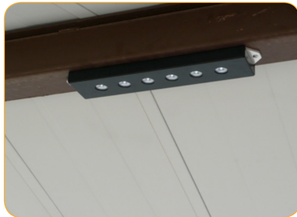
figure 7. Strip luminaire – mounted on ceiling beam
