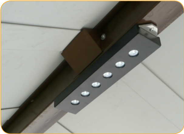
figure 3. LED Luminaire assembly (installed)
