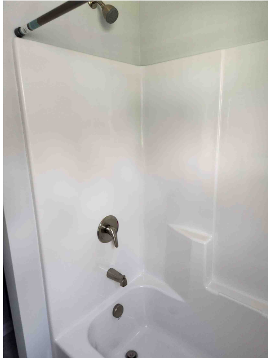
ADDITIONAL VIEW OF BATHROOM
