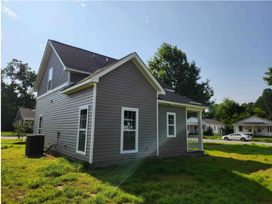
ADDITIONAL REAR / SIDE VIEW
