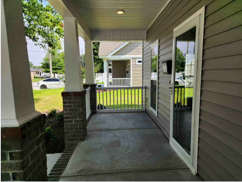
FRONT COVERED PORCH
