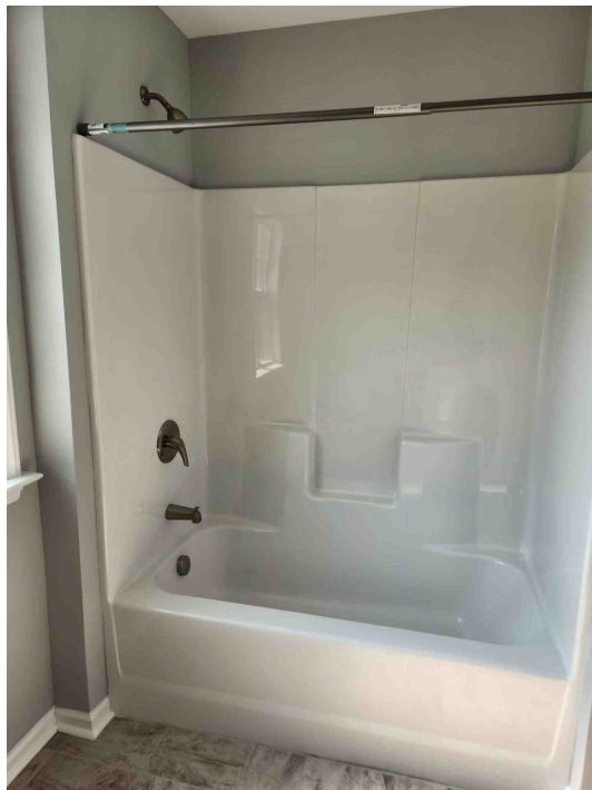
ADDITIONAL VIEW OF BATHROOM
