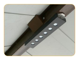
figure 3. LED Luminaire assembly (installed)
