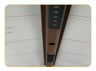
figure 6. Strip luminaire – mounted on ceiling beam
