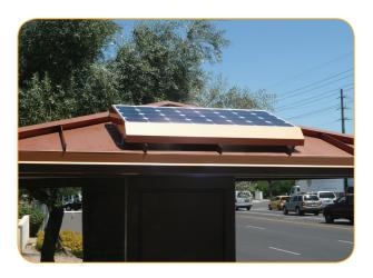
figure 2. Power module mounted on shelter
