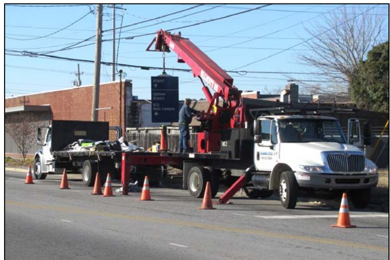
Wayfinding contractor installing new directional signs near Greenville's Airport
