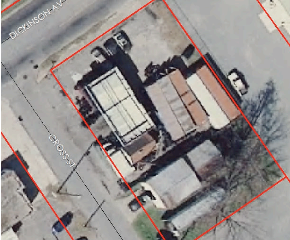
Photo #10:2012 Aerial Photograph of Dickinson Ave. Auto and Tire Source: 2012 City of Greenville, NC GIS Aerial
