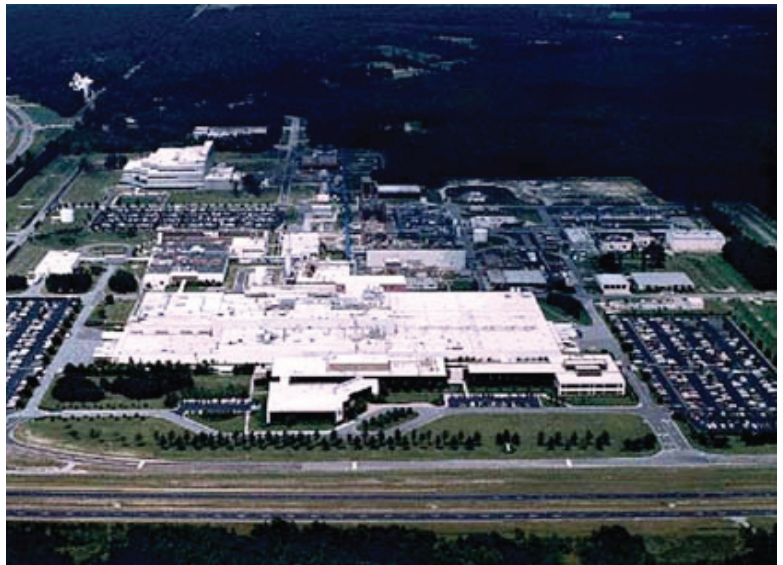
DSM Pharmaceuticals and DSM Dyneema Plant, Greenville, NC
