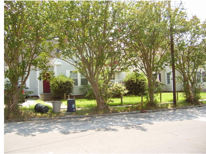
Residential structures south of 9 th St..
