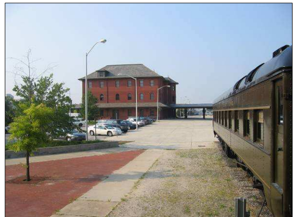
(g) Rail station, seen from bus station
