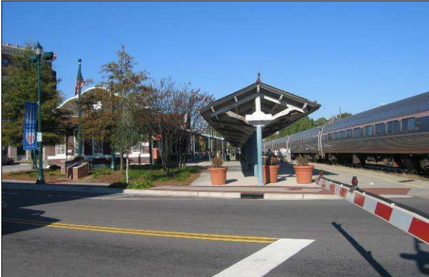
(e) Amtrak station
