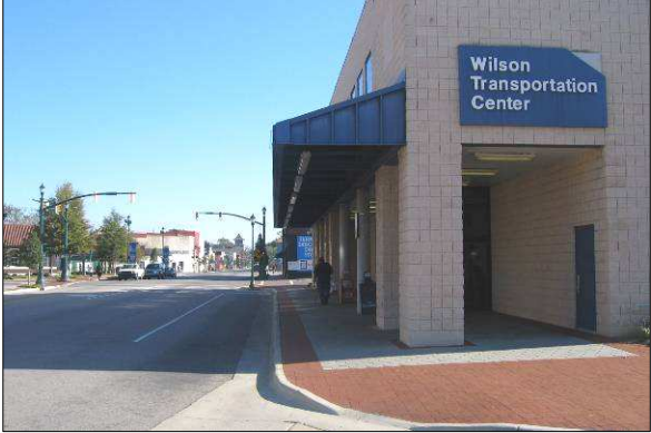
(b) Buses stop on the street. Amtrak station in left background.
