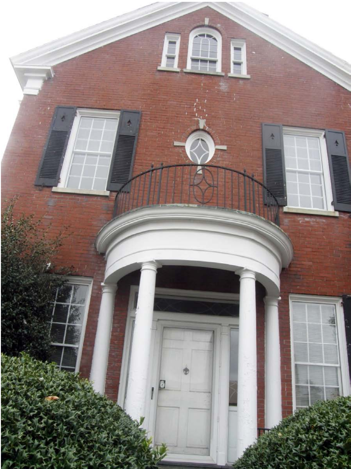
Photograph #7: North Wall Detail
