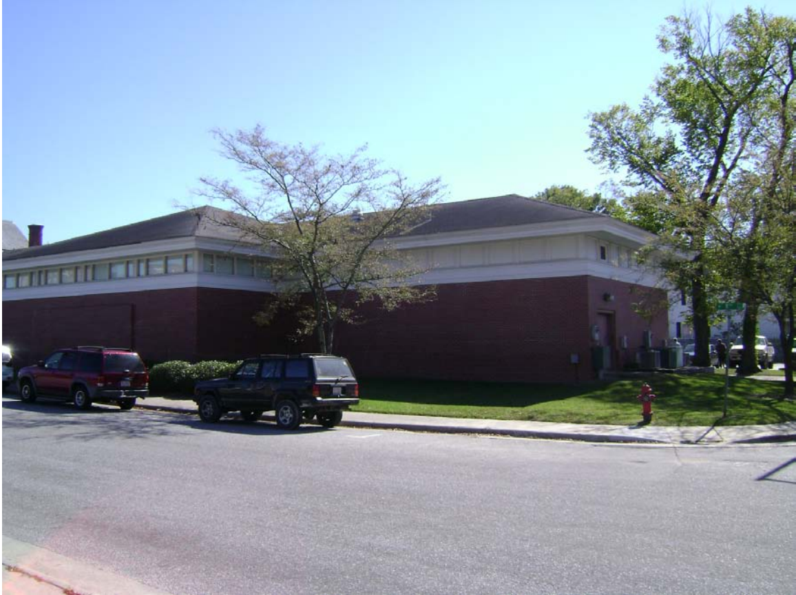
Photograph #3: Northeast Elevation (Corner of 8 th Street and Washington Street)
