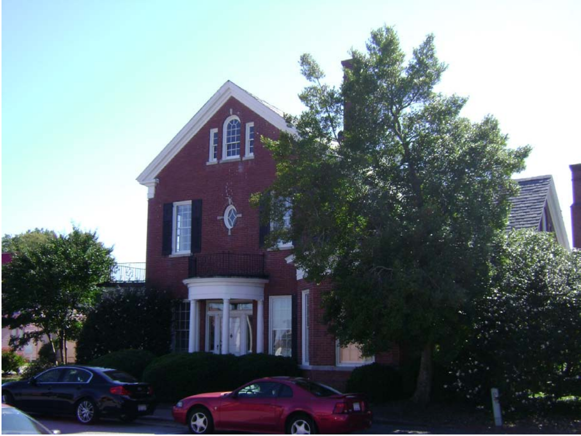
Photograph #2: North Elevation (Facing 8th Street)
