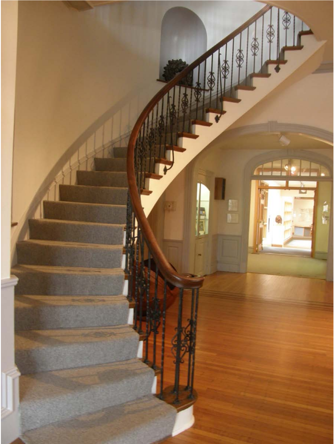
Photograph #8: Spiral Stair Detail
