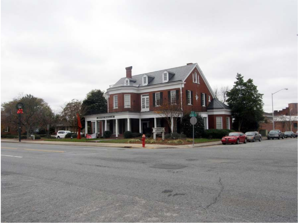
Photograph #5: Overall Northeast Corner View
