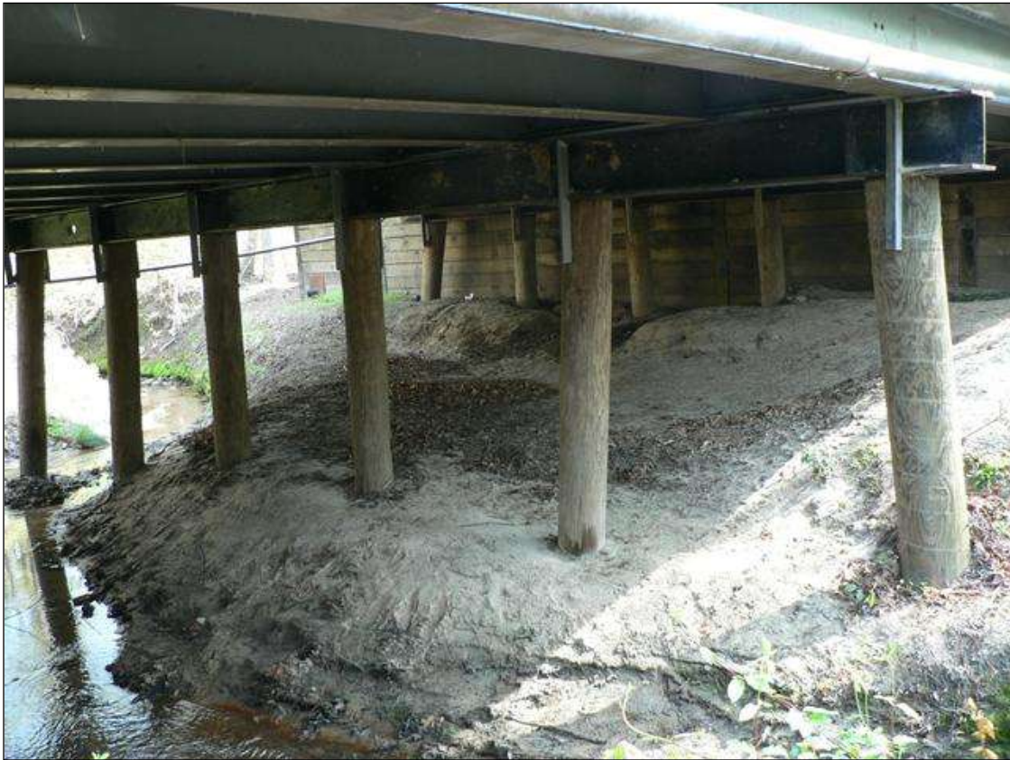
BENT, LOOKING NORTHEAST
