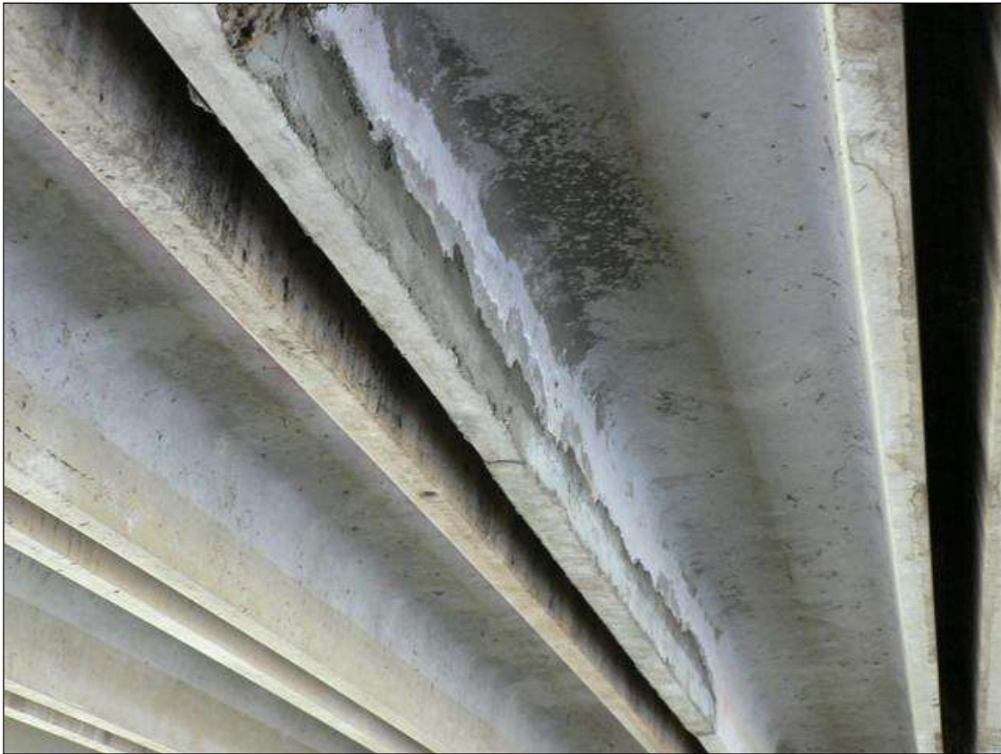
REPAIR TO LEG 1 IN CHANNEL 6 AT MIDSPAN
