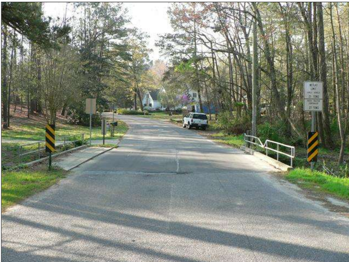
NORTH APPROACH, LOOKING SOUTH
