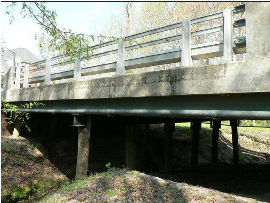
UPSTREAM PROFILE, LOOKING NORTHWEST
