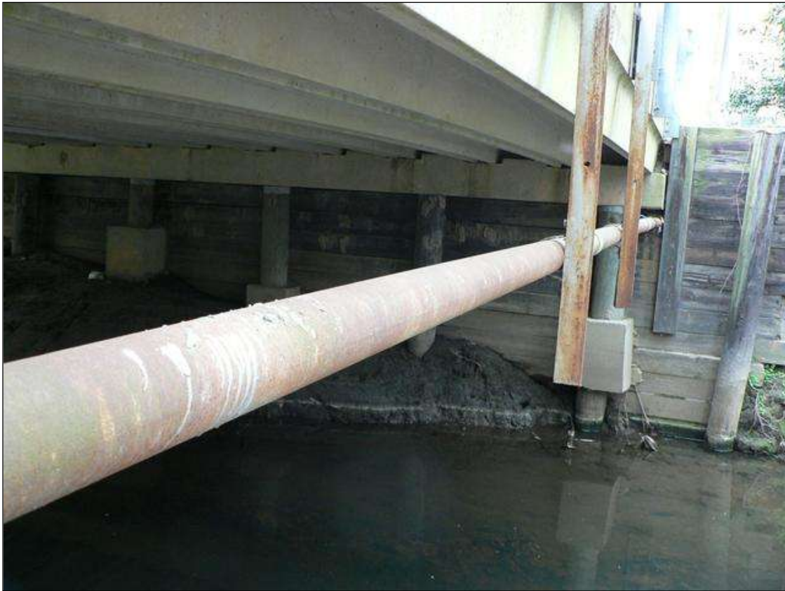
3 1/2" DIAMETER STEEL UTILITY LINE ON DOWNSTREAM SIDE
