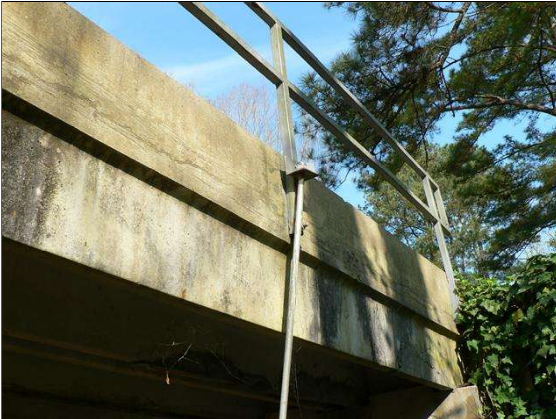
RAIL POST AND 9" DIAMETER STEEL UTILITY LINE ATTACHMENT TO DOWNSTREAM SIDE
