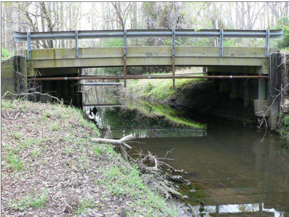
DOWNSTREAM PROFILE, LOOKING WEST
