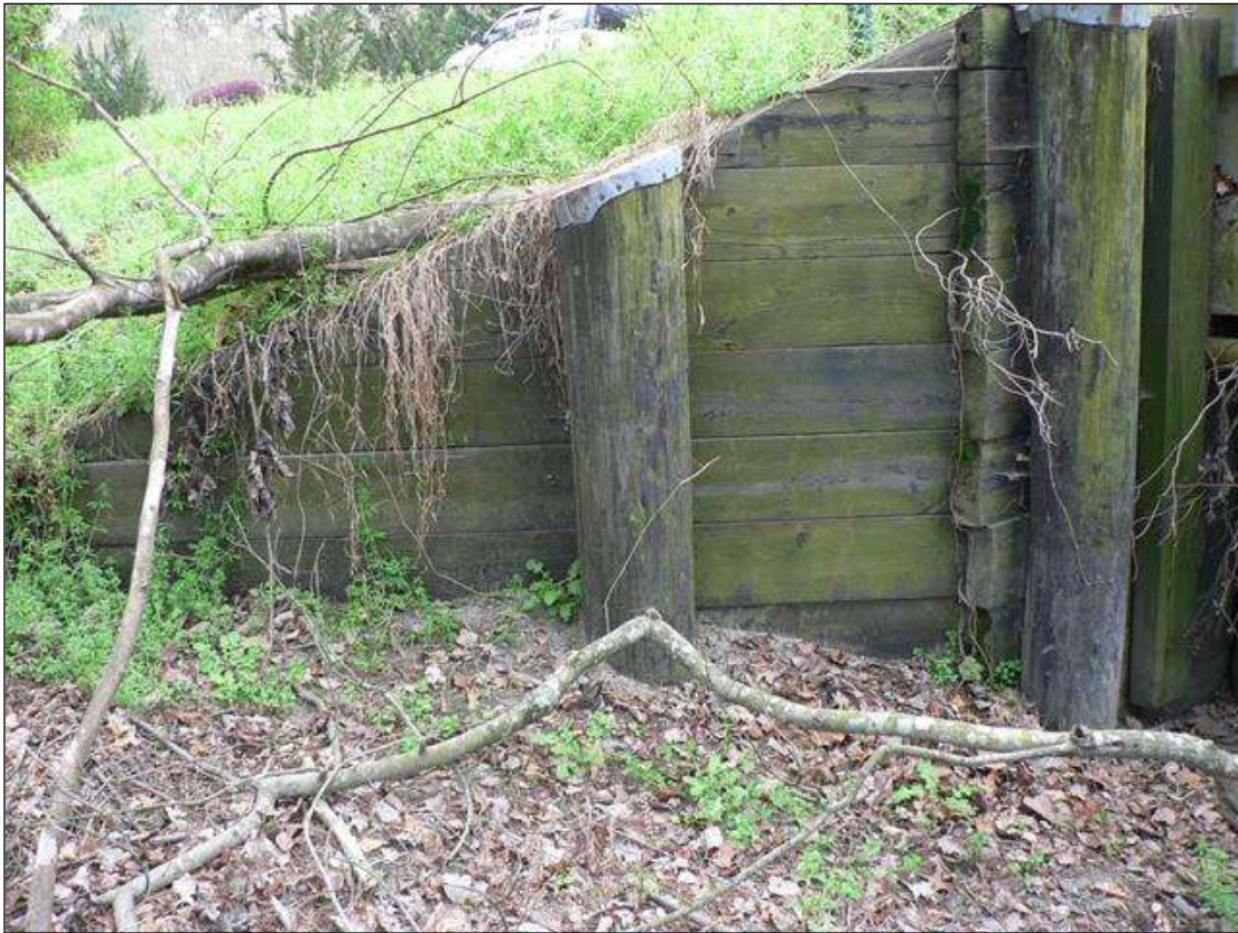
SOUTHWEST WINGWALL, OTHERS SIMILAR
