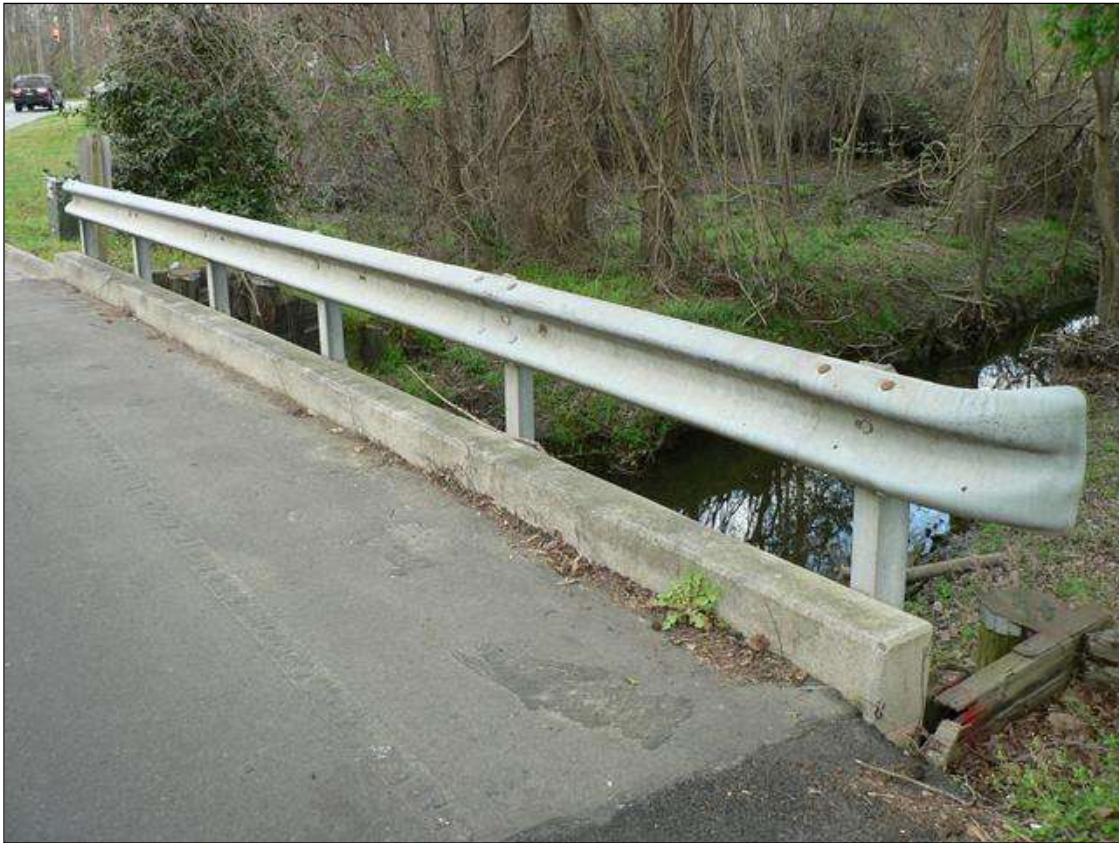
DOWNSTREAM RAIL, UPSTREAM RAIL SIMILAR
