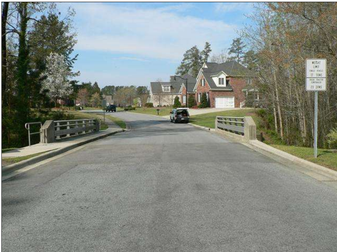
EAST APPROACH, LOOKING WEST
