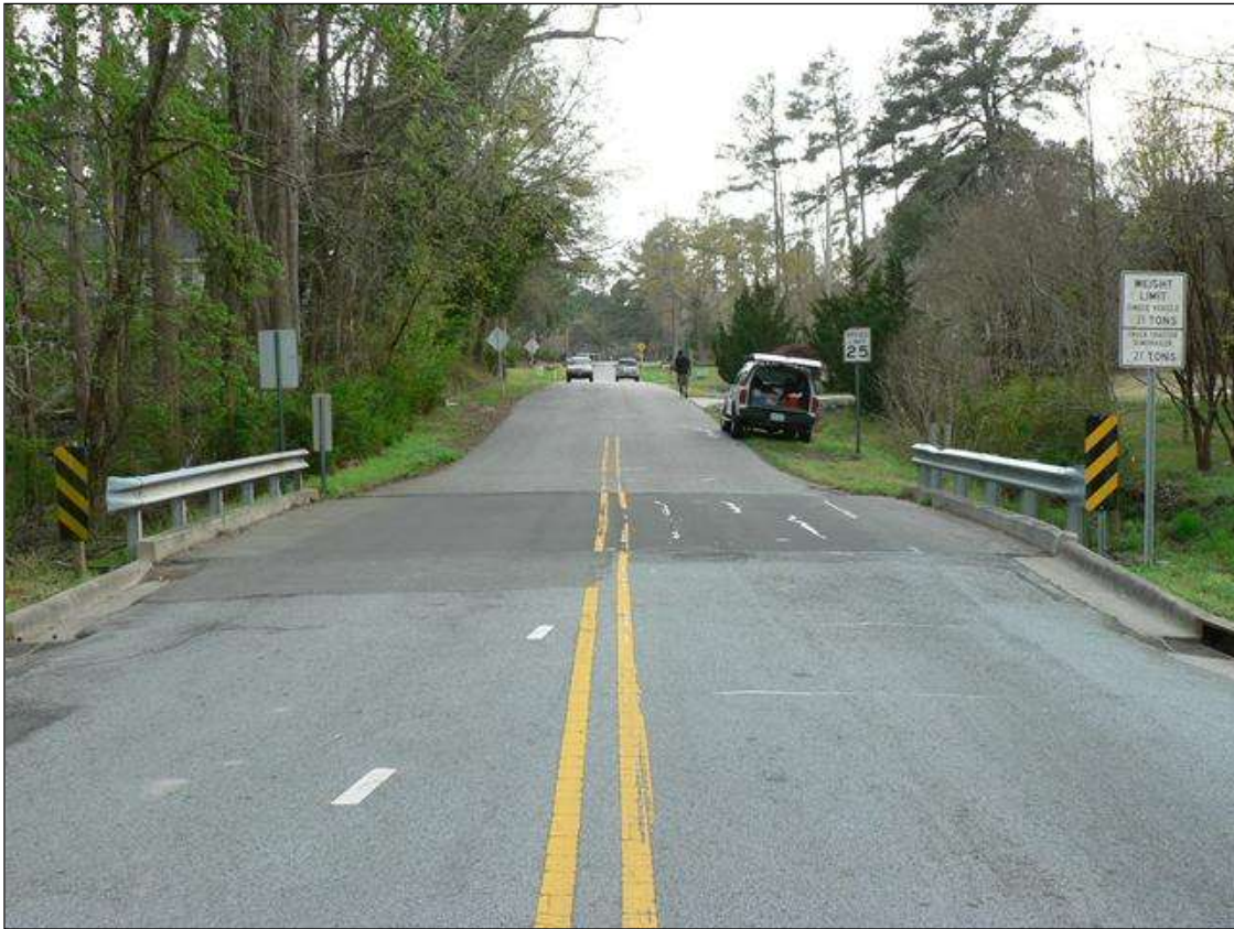
NORTH APPROACH, LOOKING SOUTH
