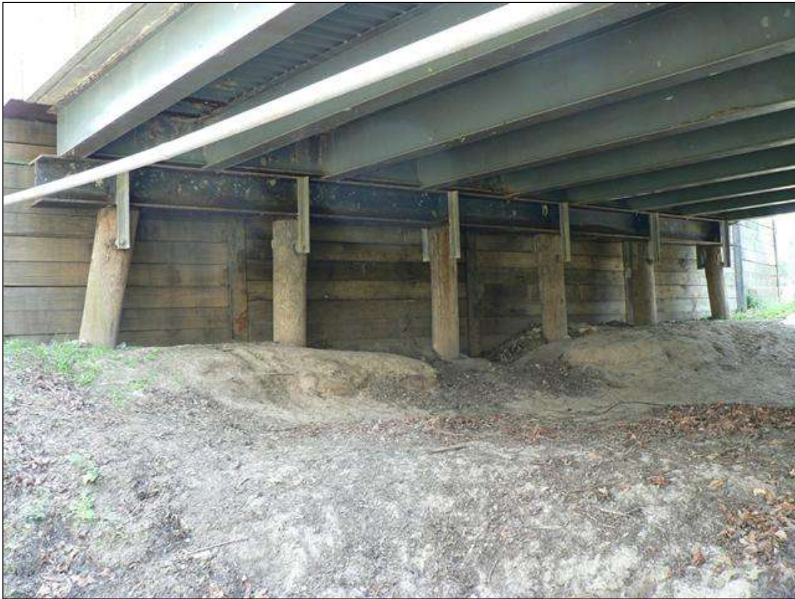
END BENT 2, END BENT 1 SIMILAR
