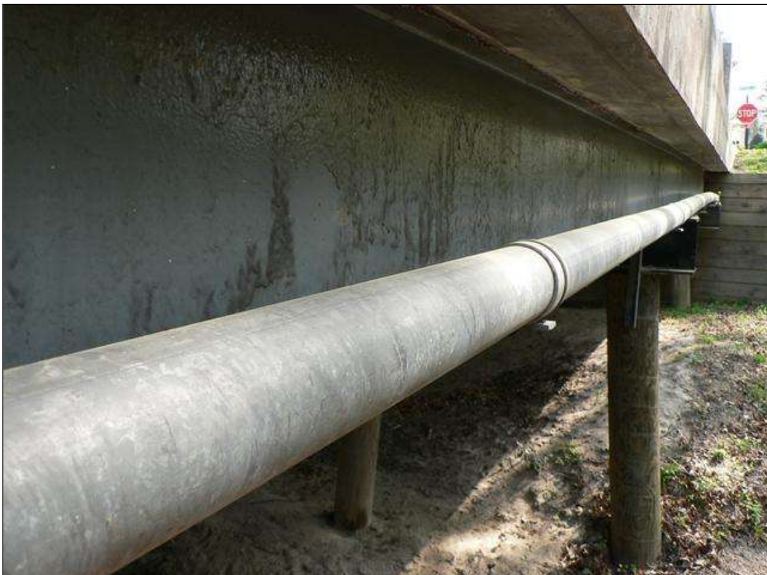
5" DIAMETER STEEL UTILITY LINE ON UPSTREAM SIDE
