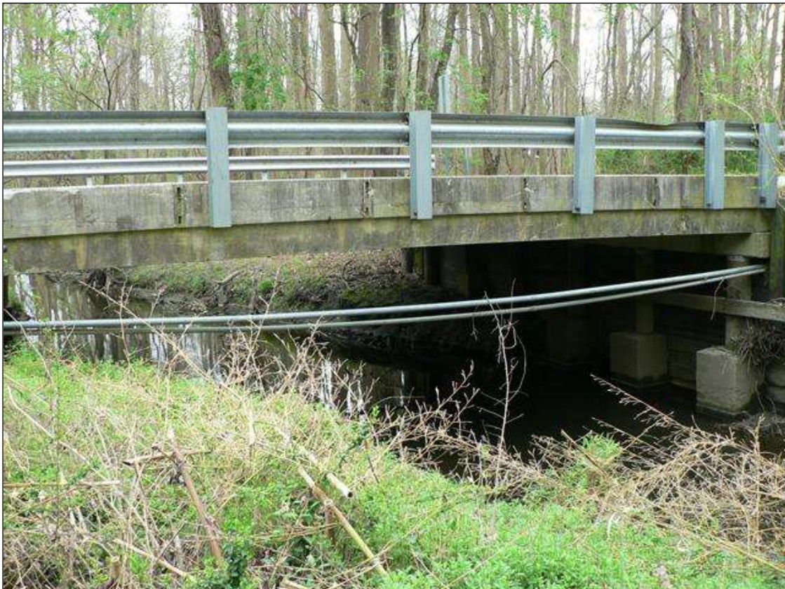
UPSTREAM PROFILE, LOOKING SOUTHEAST
