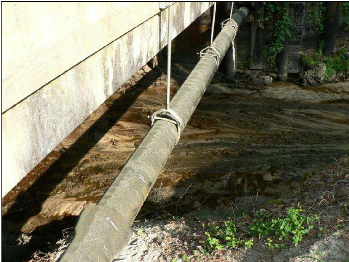
9" DIAMETER STEEL UTILITY LINE ATTACHED TO DOWNSTREAM SIDE
