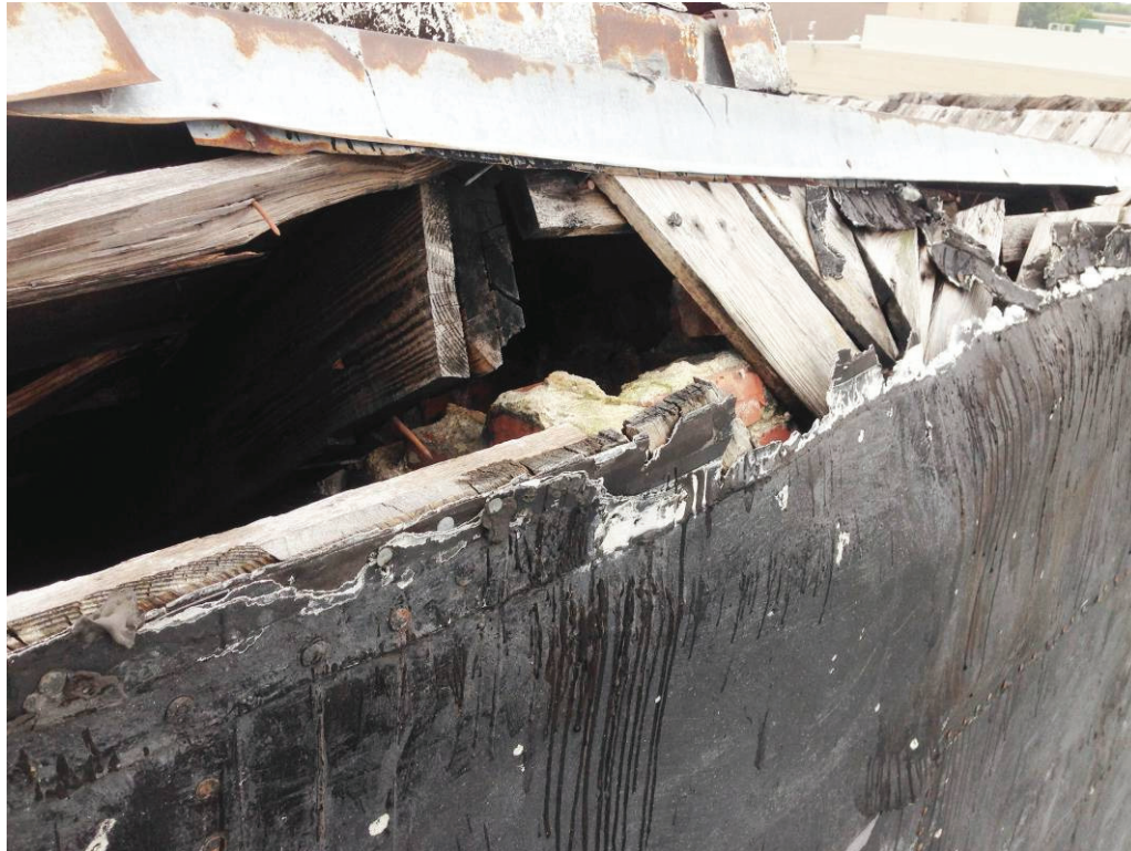
Photograph 4 – Chimney Damage
