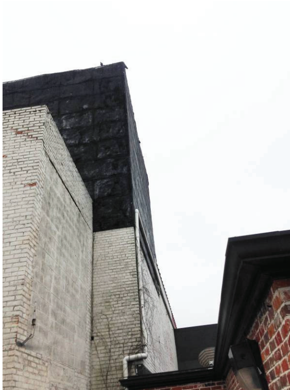
Photograph 5 – Fly Loft Right Side Wall
