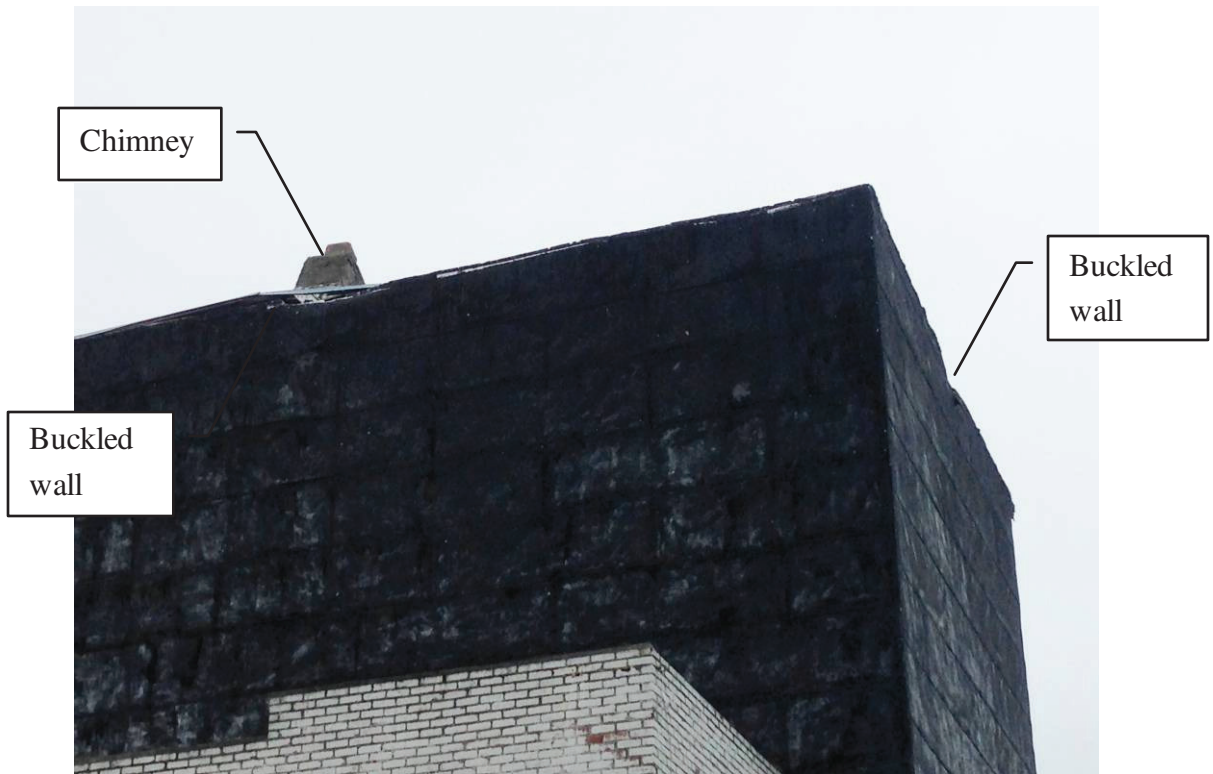
Photograph 1 – Leaning Chimney and Buckled Walls at Rear of Fly Loft Area
