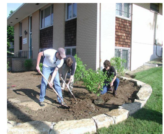
Installation of a traditional rain garden.
