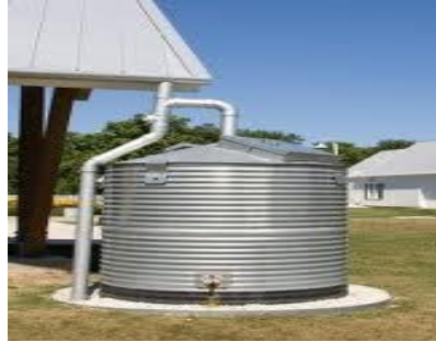
Rain barrels or cisterns can store rain water for irrigation or wash water for vehicles.
