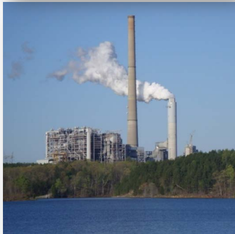
Mayo Plant 16.17% Ownership (118 MW)
