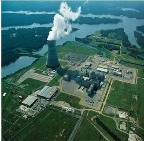
Harris Plant 16.17% Ownership (146 MW)
